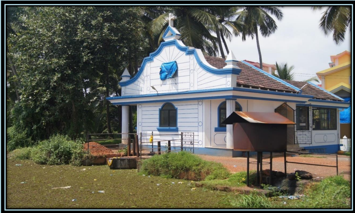
HANDI CROSS AT MAINA AND SLUICE-GATE
