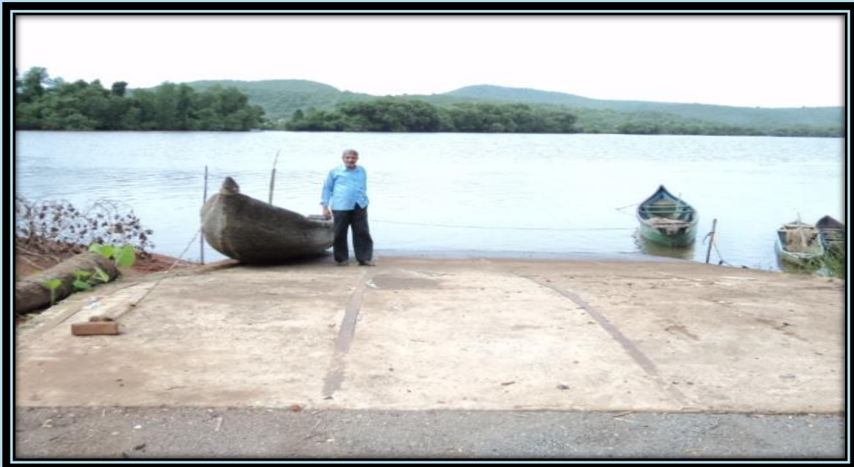
RAMP AT ULLANDO
